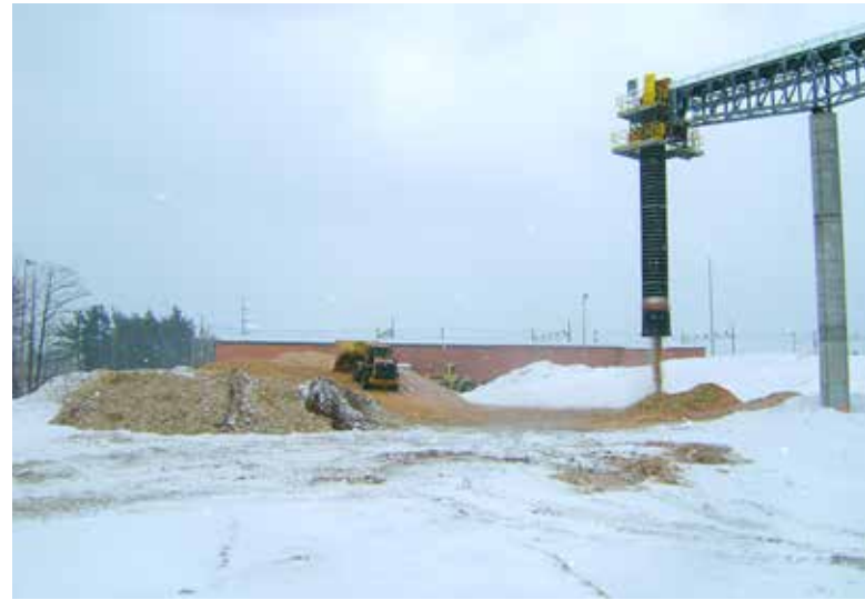
The fuel pile being built by the 70-foot telescoping chute.
